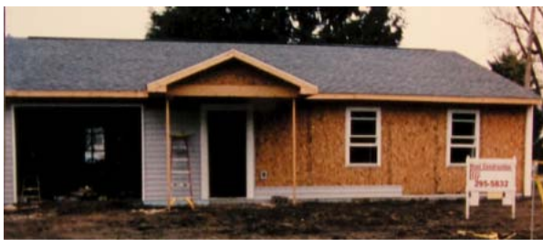
Vannoy's Partially Completed House.
