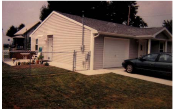
Vannoy's Handicapped Accessible House: Completed and Now a Home.
