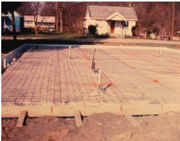
Slab for Vannoy's Accessible House.
