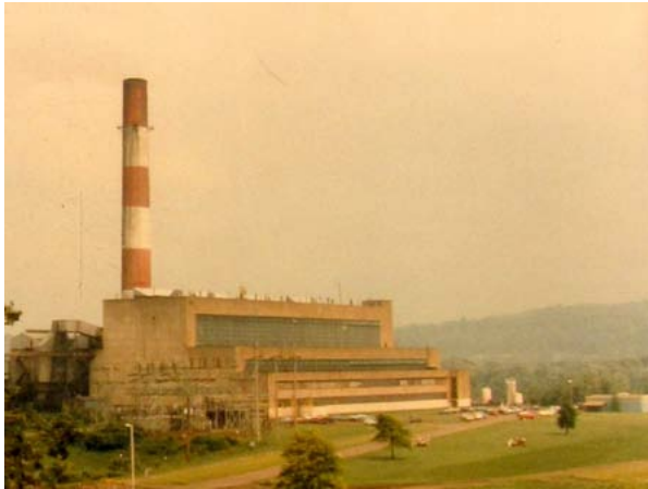
Outside of Gorsuch Plant--Notice the Height of the Plant.
